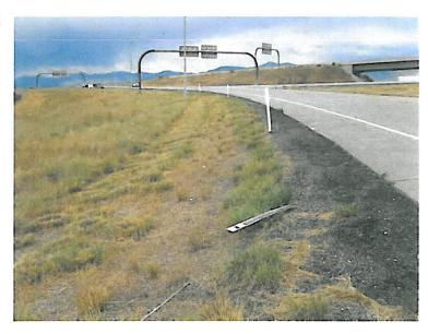
For areas where delineators are frequently damaged, the lower life cycle cost of the SHUR-TITE delineator amounts to an annual savings of \$75 per installation. Traffic services are improved because delineators remain serviceable, risk exposure of UDOT employees is reduced due to fewer service calls, and less scrap materials requiring disposal are created.
